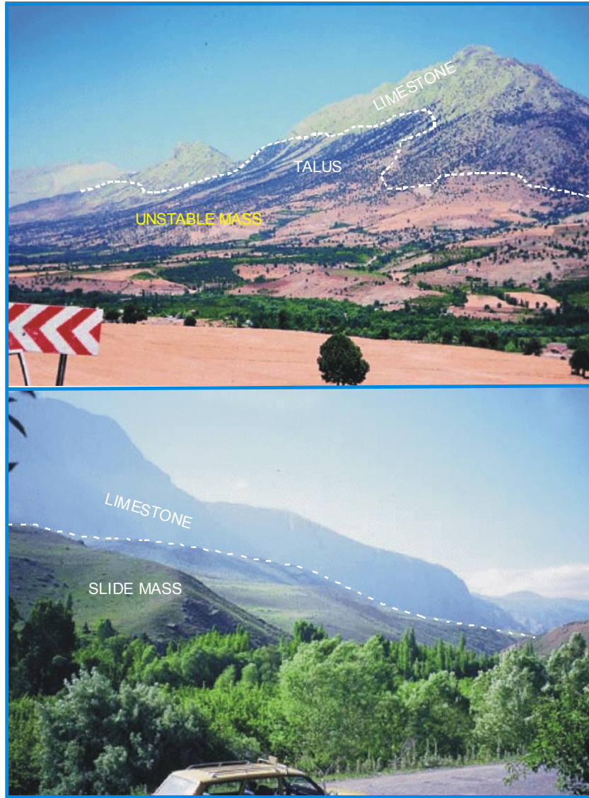
Figure 2. Slide masses in Ecemiş Fault Zone.
