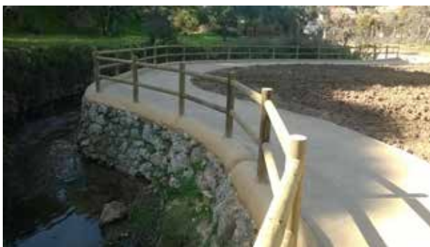
Figure A13 Ribeira das Vinhas greenway restoration project
