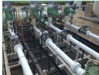
Sentinel LCT4 or LCT8 4 and 8 path liquid meters for the above mentioned applications.
