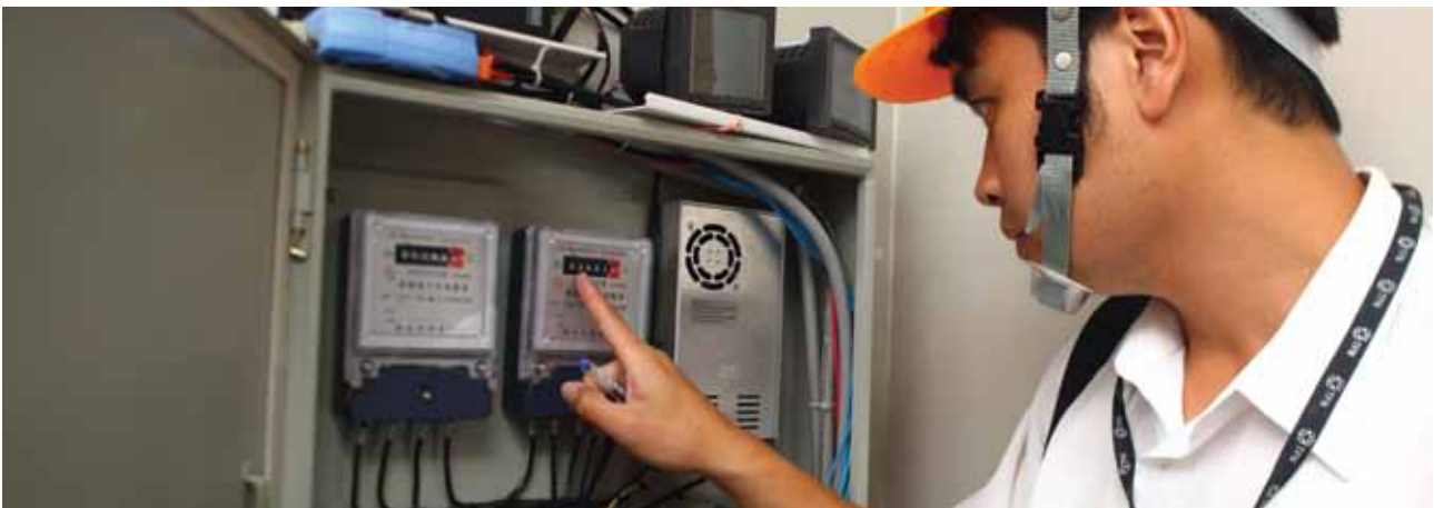
▲ We have installed high-efficiency, low power consumption, precision air conditioning systems at our 3G base stations.
