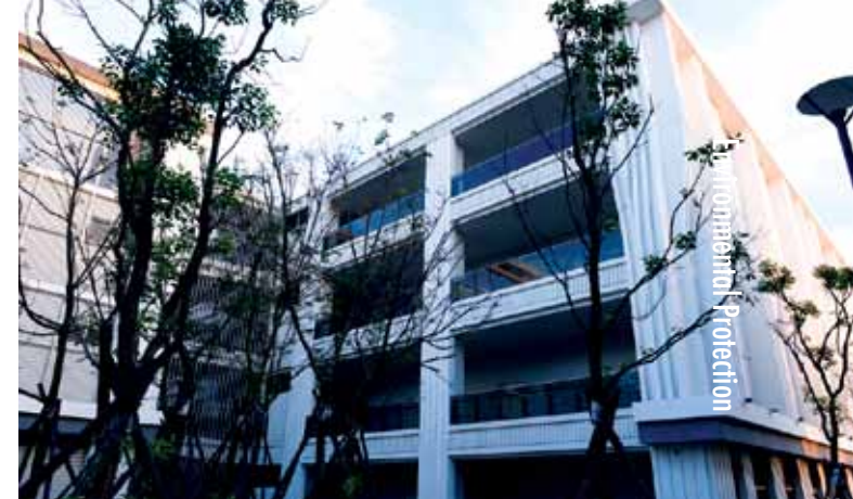
A new green cloud data center is the first one in Taiwan to receive an Uptime Institute Tier III certification.
