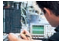
MAINTENANCE OF CONTROLS
