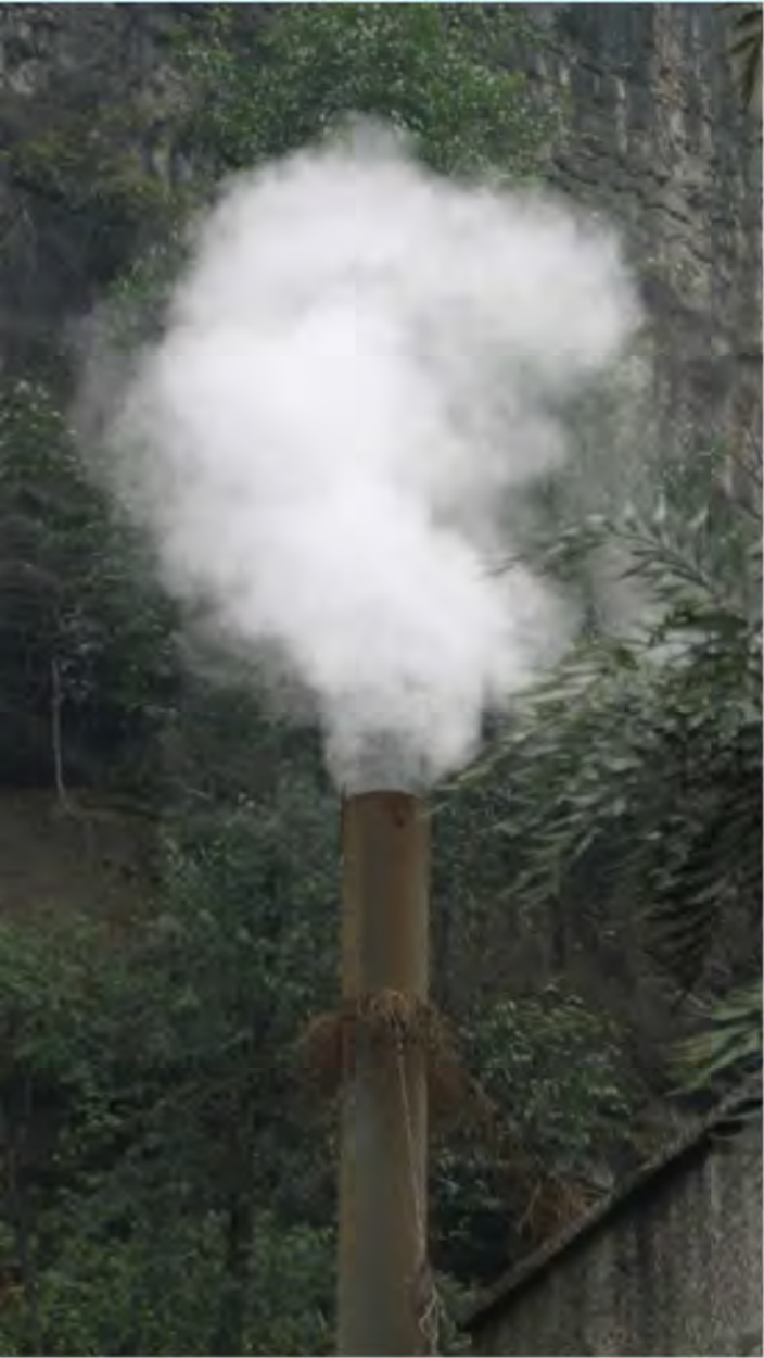
CMM escaping through a vent stack
