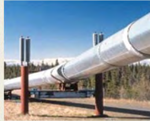
Pipeline Injection/ Town Gas
