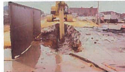
2. Construction of Slurry Wall
