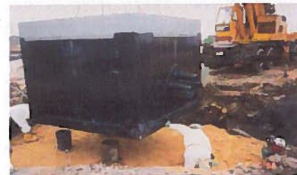
3. Head Maintenance System Component Installation
