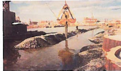
1. Construction of Stone Embankment
