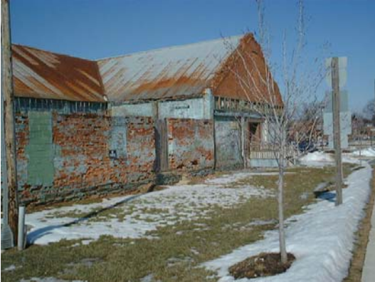
East Street Façade of Lippart's Cabinet
