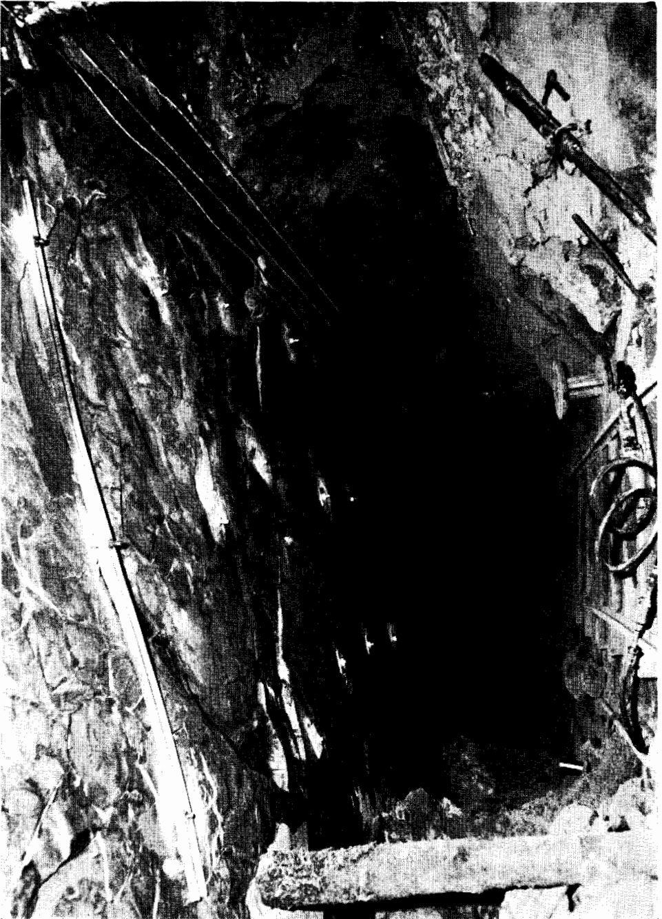
Big Savage Refractories Corporation—Section showing new method of Roof Bolting
