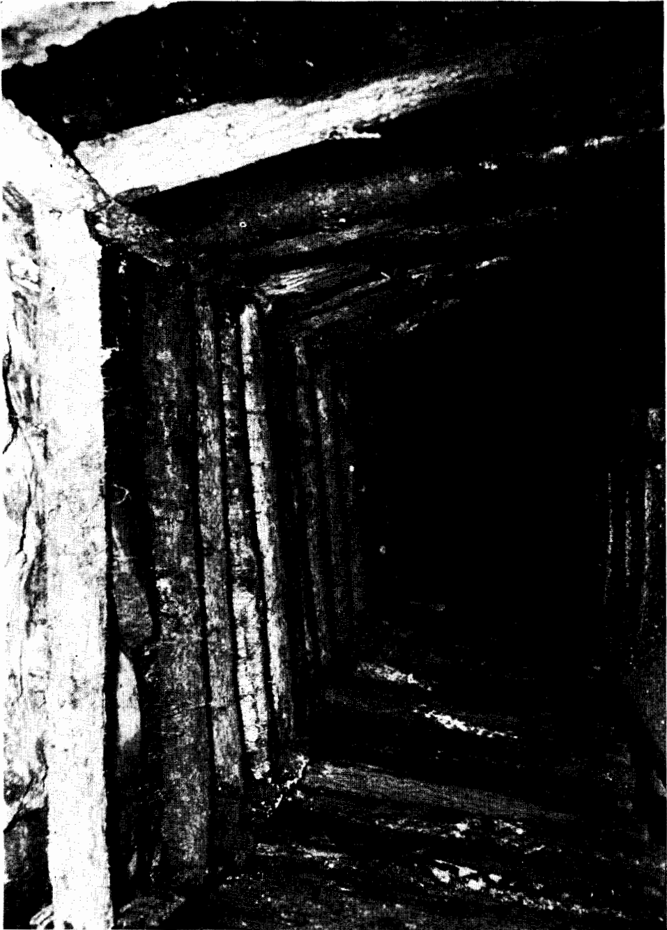
Big Savage Refractories Corporation—Section showing old method of timbering
