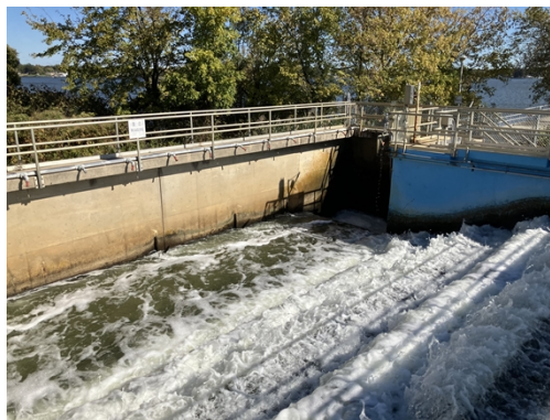
Image 04: Step Aeration system, final effluent.
