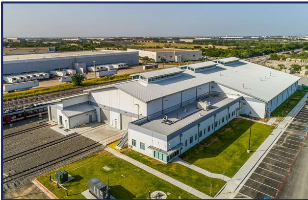
Mahaffey Maintenance Facility (MMF)
