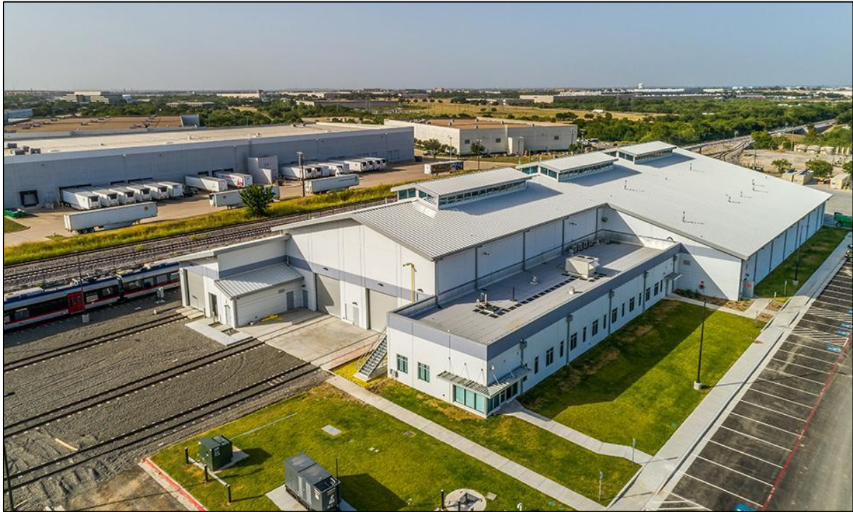
TEXRAIL Mahaffey Equipment Facility, Fort Worth, TX. Photo courtesy of Huitt-Zollars, Inc.
