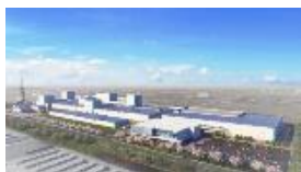
Hitachinaka Factory (Ibaraki) (Under construction)
