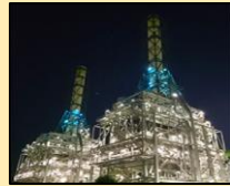
▲ Kawasaki Natural Gas Power Plant
