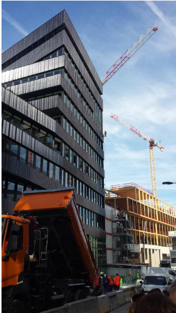
Blocks under construction in Clichy-Batignolles, May 2017.
