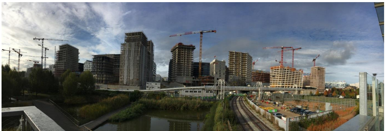
Panoramic view of the CoRDEES blocks under construction. Author: Juan Cuevas.
