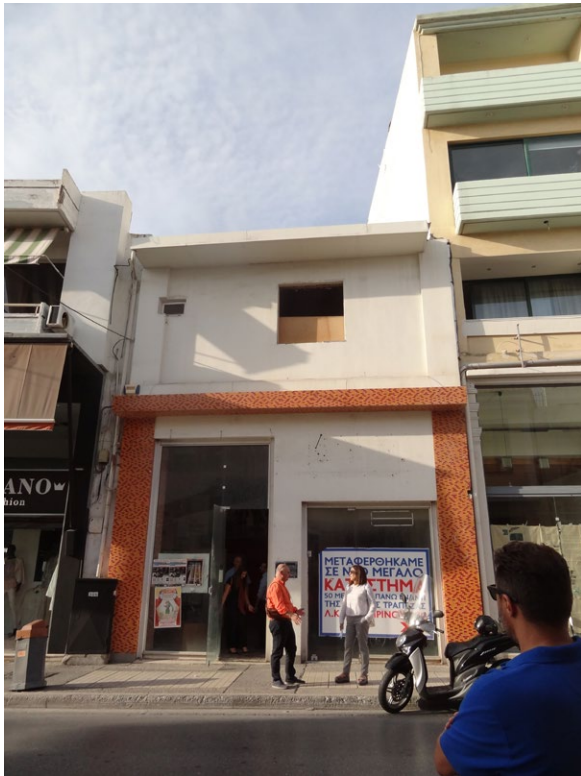
The building that was selected for the Second Opportunity Restaurant
