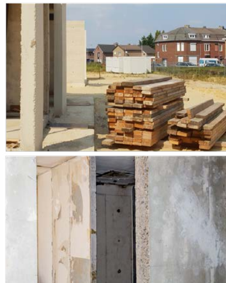
Figure 4: Main building materials recovered from the high-rise social housing building from 60's and reused by remanufacturing
