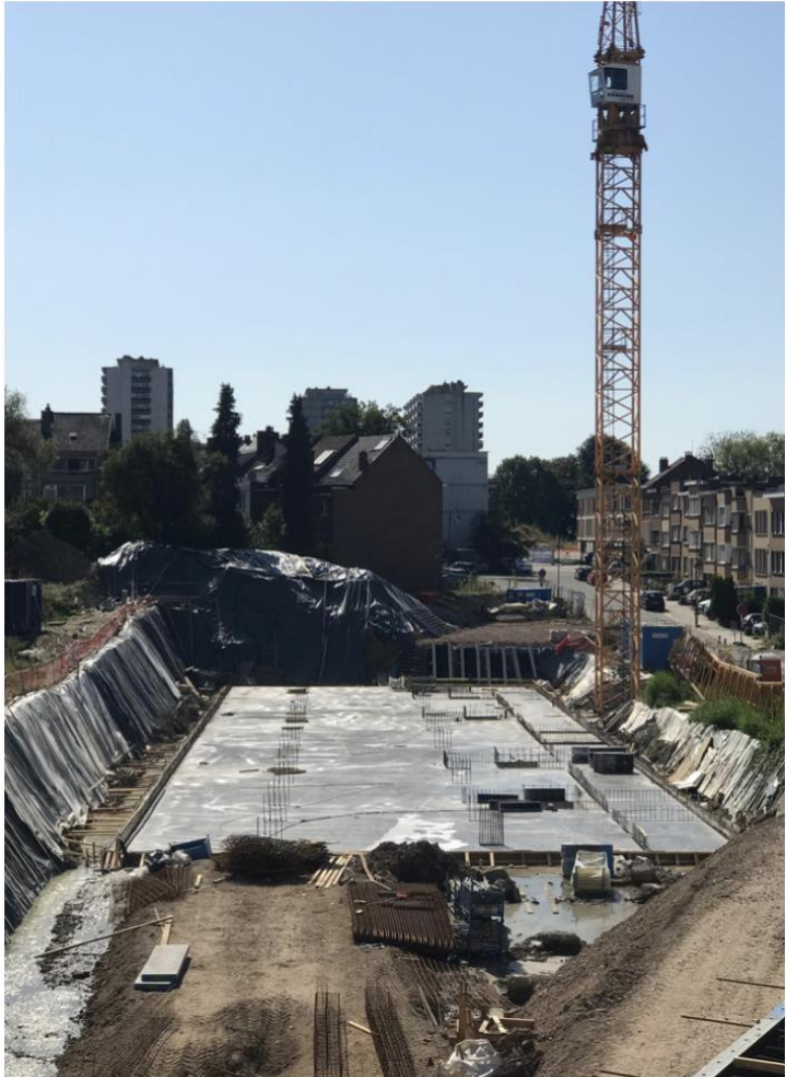
Figure 11: CALICO site under construction. Source: I Verbist.
