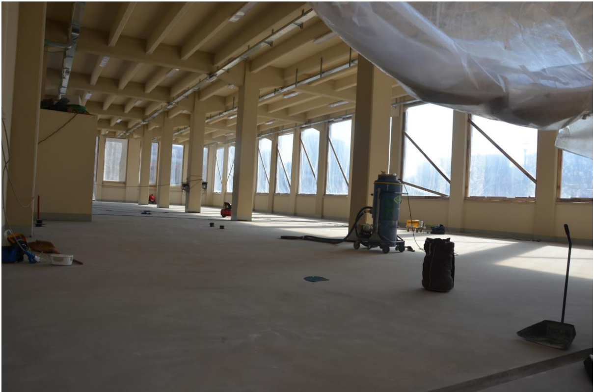
Figure 3 Via Cumiana structure. Source: site visit on February 13, 2020)
