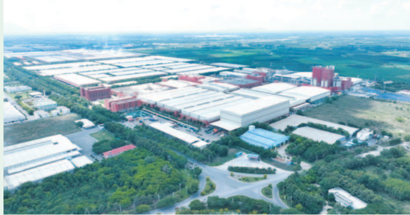
Phuoc Dong Industrial Park, Go Dau district, Tay Ninh province is an attractive investment destination
