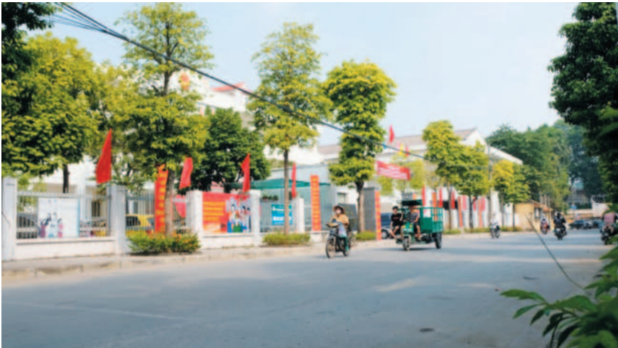
Gia Lam district's infrastructure is continuously upgraded to support both residents' needs and economic growth
