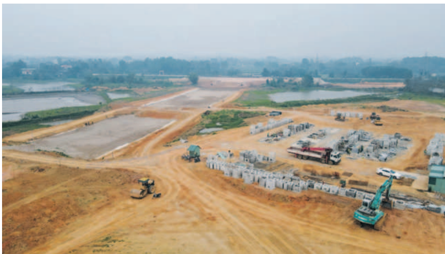
Song Lo II Industrial Park is accelerating construction progress
