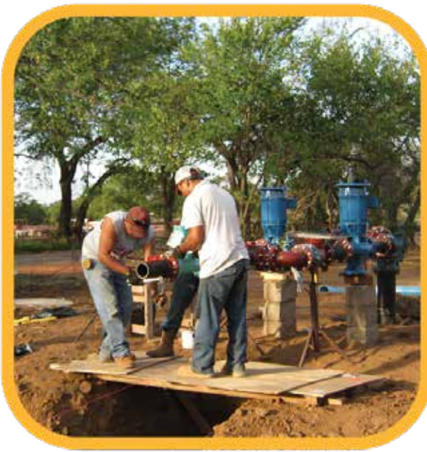
Pump station construction in progress
