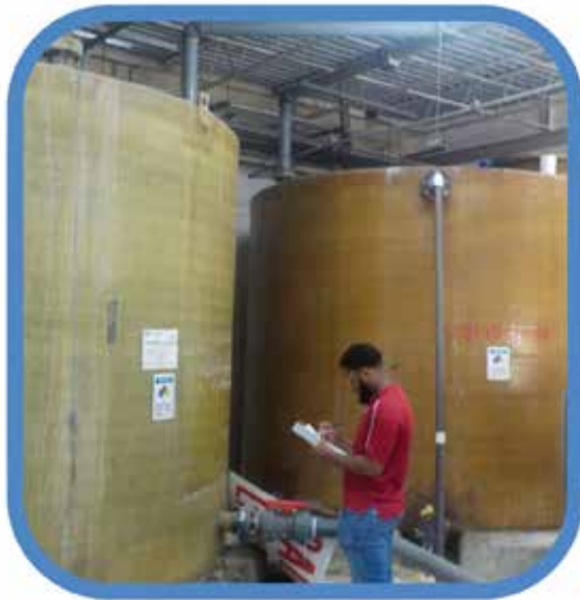
Engineer Xavier Branch conducting a bulk chemical storage tank inspection during a sanitary survey.
