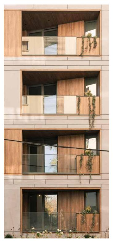
Our Max Compact panel has a green core and consists of around 65% paper as a carrier material. We already cover half of this core paper requirement with 100% recycled paper. The remaining paper comes entirely from sustainable forestry and is FSC and PEFC certified.
