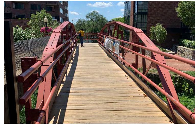
5 33RD STREET NW AT M STREET
