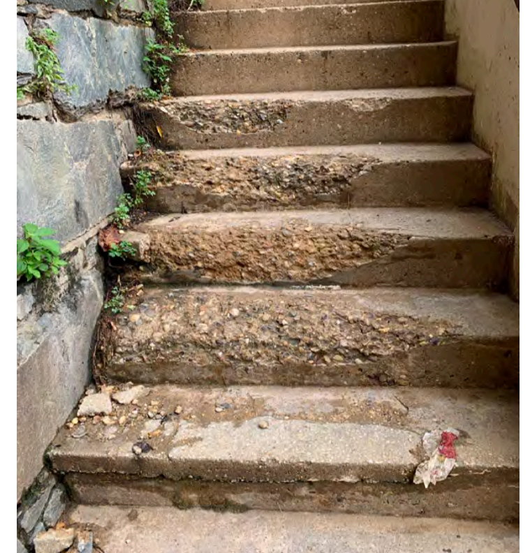
CONCRETE STAIRS FROM C&O CANAL
