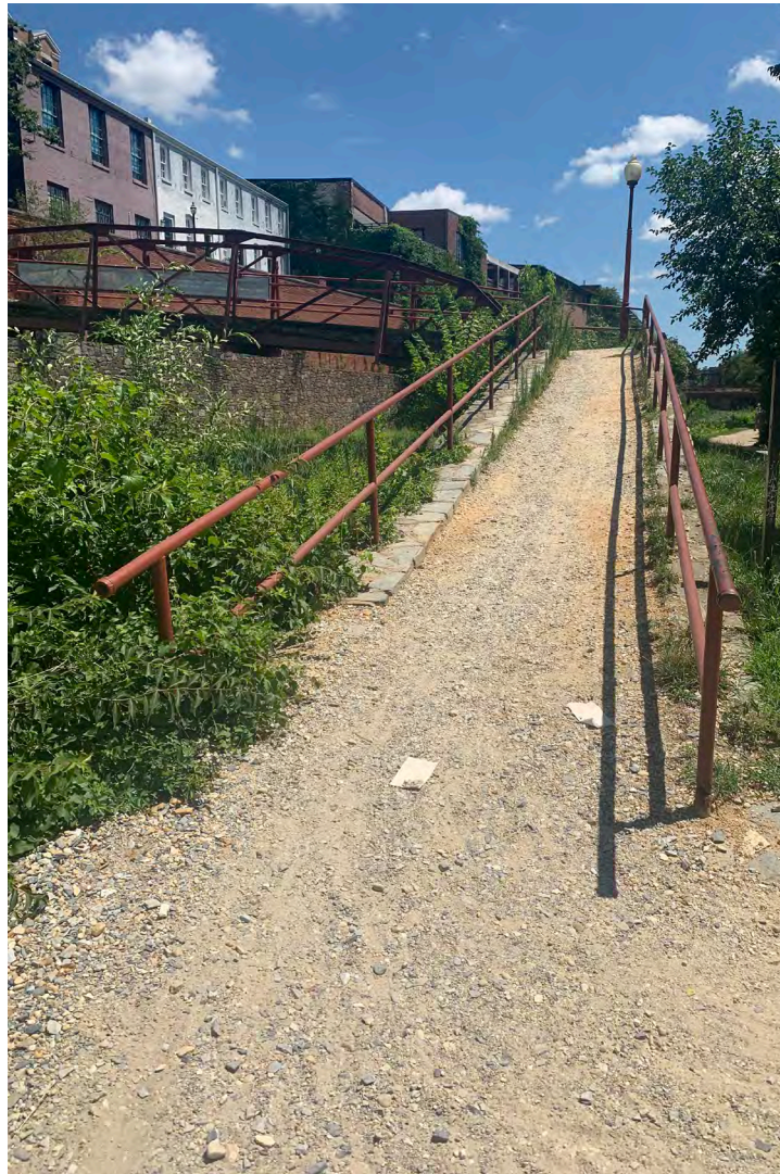
2 34TH STREET BRIDGE
