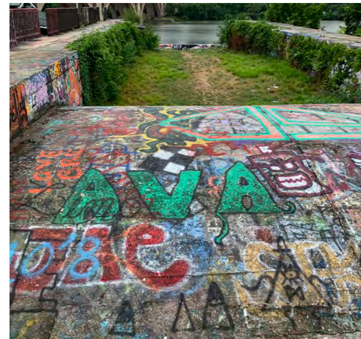
GRAFFITI AT ALEXANDRIA AQUEDUCT
