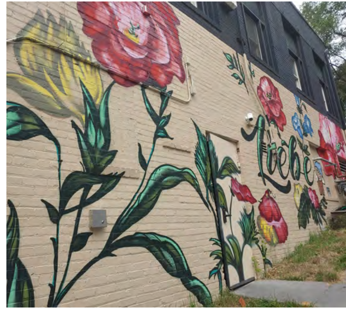
WALL TREATMENT ALONG K STREET AT THE BERLINER
