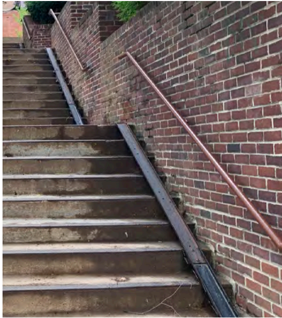
ACCESSIBLE BIKE RAIL AT 34TH STREET NW CONNECTION TO CANAL
