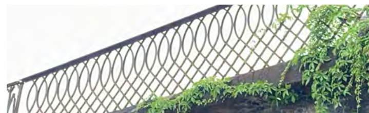
ORNAMENTAL RAIL AT ALEXANDRIA AQUEDUCT
