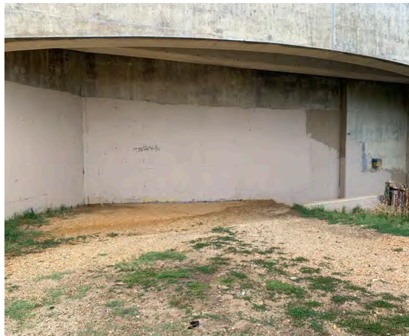
THRESHOLD FROM C&O CANAL TO TRAILHEAD SITE
