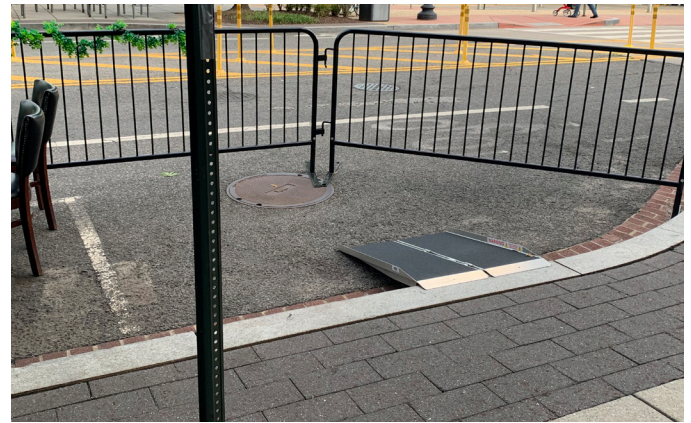
TEMPORARY ADA RAMP
