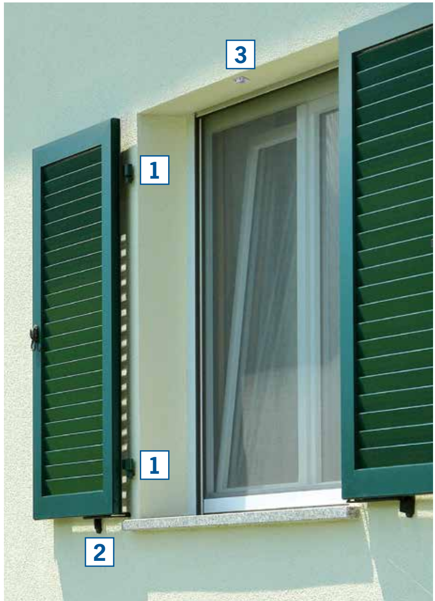
1 Fastening the clamp next to the window with support bracket K1-PE
