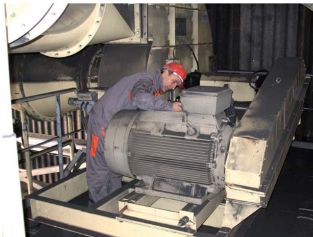
Figure 2: Execution of an energy audit
