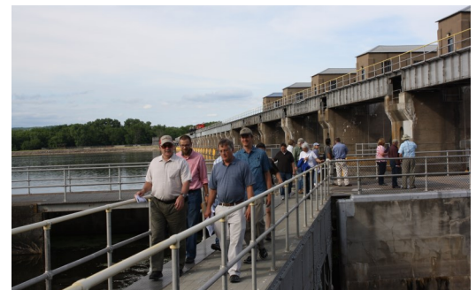
United States Army Corps of Engineer Lock and Dam Number 5, Minnesota City, invasive carp research with the University of Minnesota and Minnesota Department of Natural Resources.
