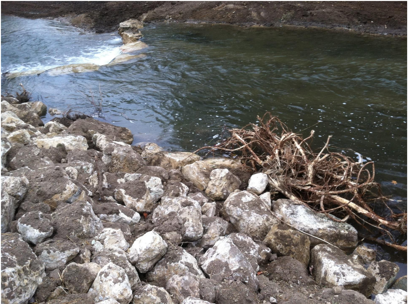
Weir and Rootwad
