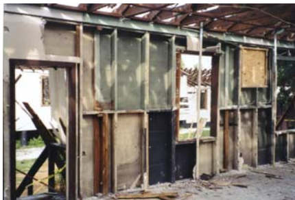
Down to the sheathing and rafters
