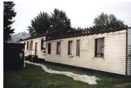
Roof has been removed
