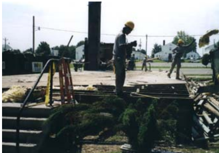
Preparing to remove decking
