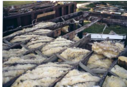
Decking removed - insulation
