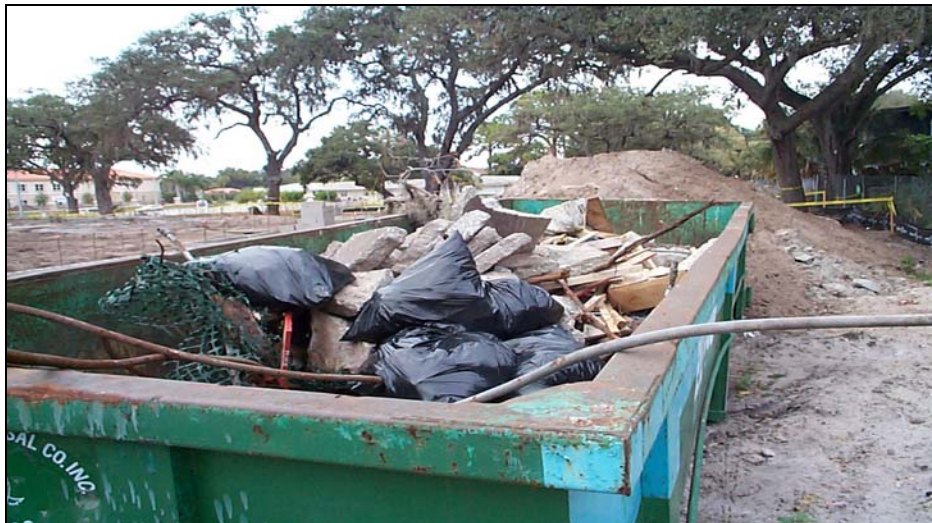
Dumpster full of C&D waste
