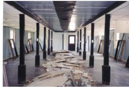
Sheetrock and Windows removed
