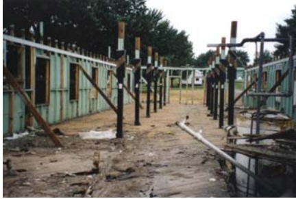
Walls secured against collapse
