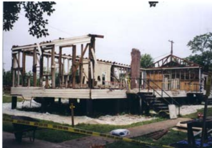
Walls and siding removed
