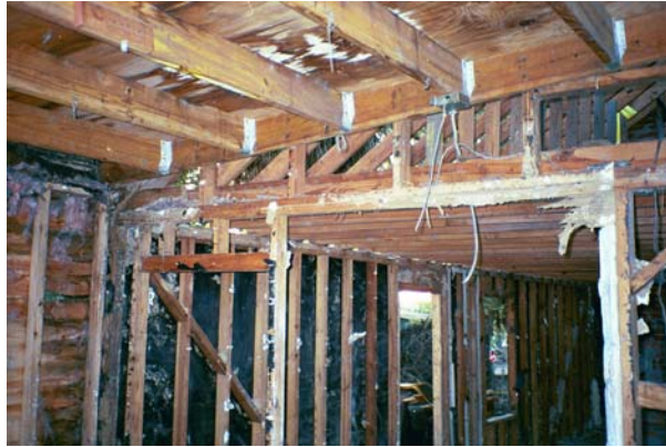
a one story building all cleaned up
