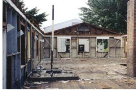
Clean and secure work area
