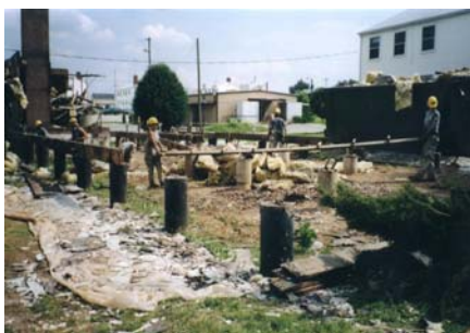
Down to the supports
