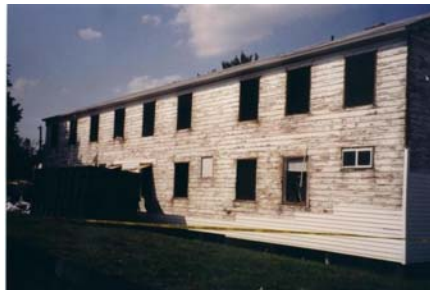
Outer siding removed
