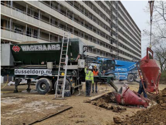
Figures 3b - Use of recycled aggregate from the existing neighbouring block for the construction of the fundaments and ground floor slab (reuse on material level/lowest level of building decomposition).
