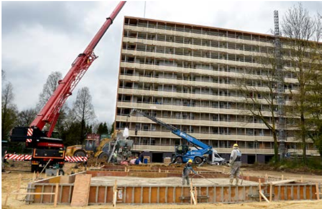
Figures 3b - Use of recycled aggregate from the existing neighbouring block for the construction of the fundaments and ground floor slab (reuse on material level/lowest level of building decomposition).
