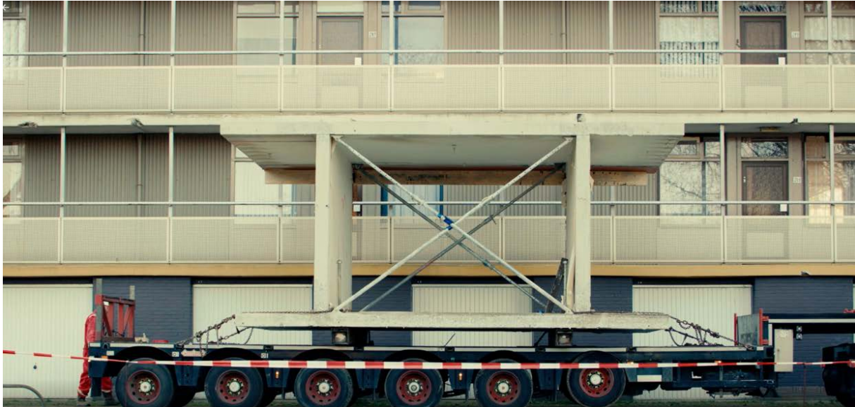
Figure 9 - high value recovery of 3D unit to be used in new SCE house
