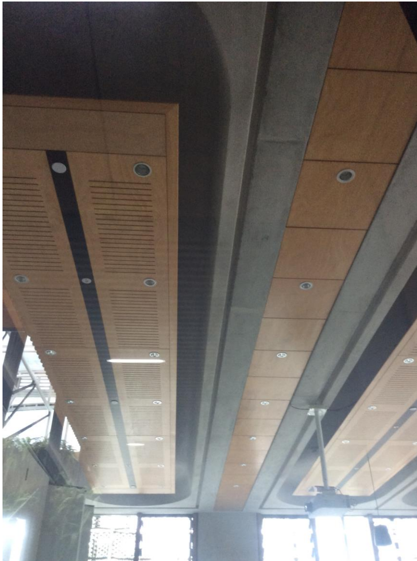
Figure 7. Queensland's University GCI building – ceilings/floor (geopolymer cement based on fly ash)
