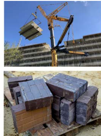
Figure 5: Restart of product life by resourcing 3D unit form the existing building otimised for one reuse
