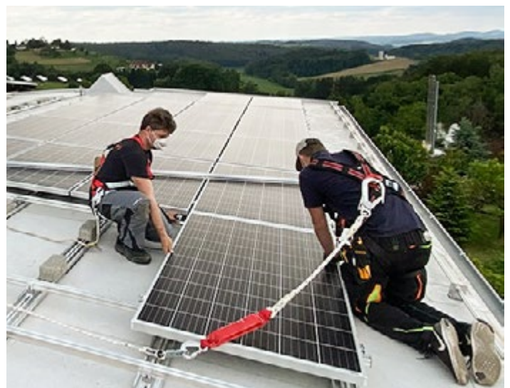
Montage neuer Photovoltaikmodule.
